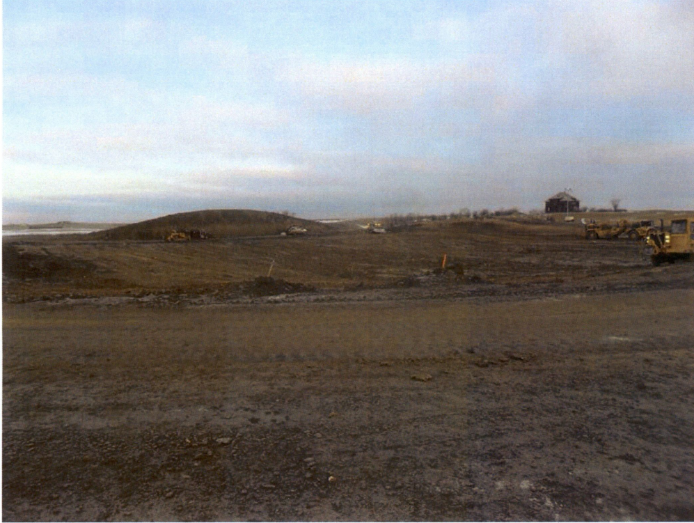
Report Photo #2 “Topsoil pile left. Subsoil pile right” at GPS Coordinates: 48.285556°N 103.322778°W
